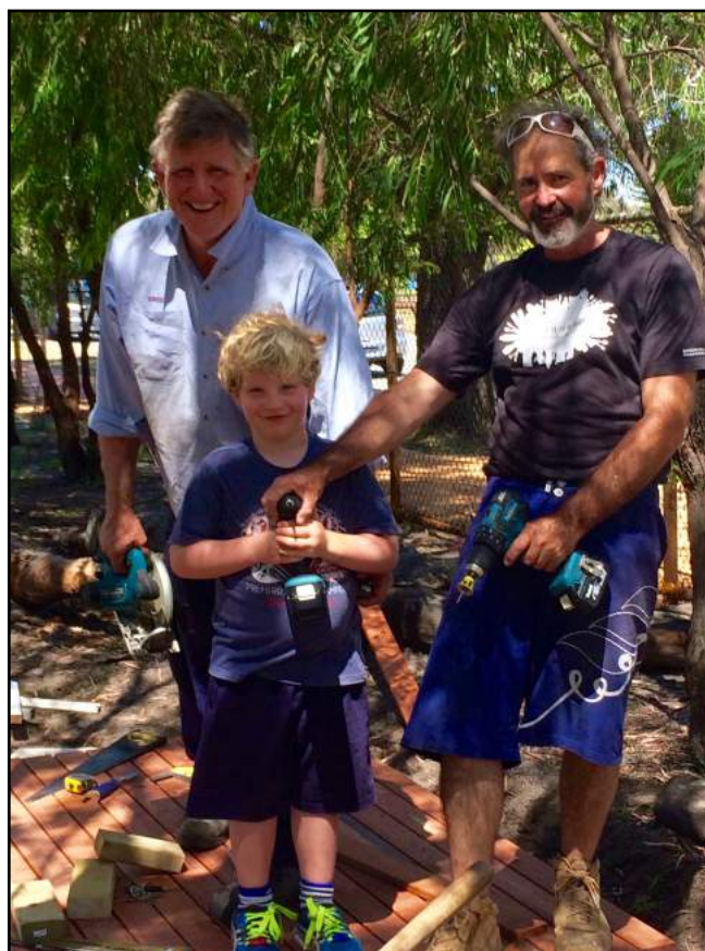
Mr Greg Finch and Mr Rob Farish pictured with Campbell putting the finishing touches on the decking.
